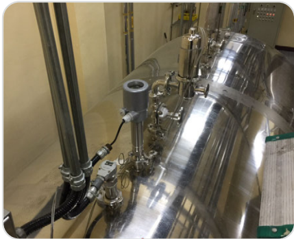
Water purification barrel
