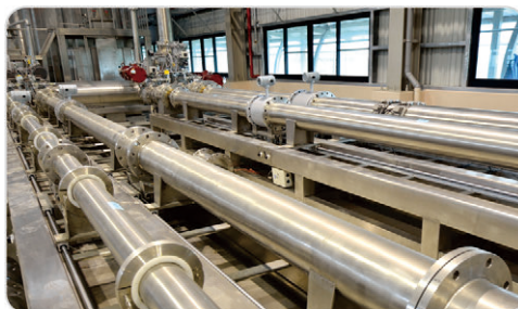
Piping system II (Maximum diameter is 300mm)
