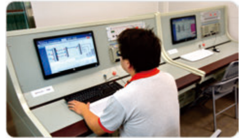
Control room & Graphical HMI
